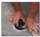
the concrete around the ½" risers. Cut the ½" PVC pipe to accommodate the proper installation of the Rain Deck housing. The ½" riser should be cut so that when the housing is installed, the top of the housing will be flush with the top of the finished surface material (ie. If ½" rubber surfacing will be applied as a surface material, set the housings ½" above the finished concrete).
