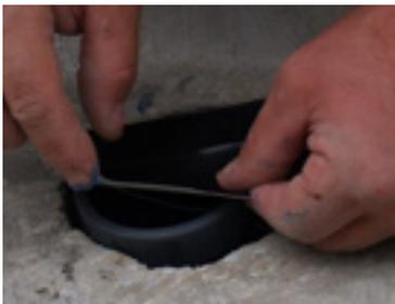
Take proper precautions to ensure concrete or other debris does not get into the Rain Deck housing.
