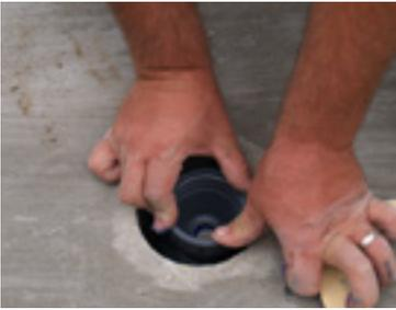
After the Rain Deck housing has been connected to the supply line, use mortar or a similar concrete product to fill the void around the housing. As the mortar sets up, use a level to ensure that the housing is level.
