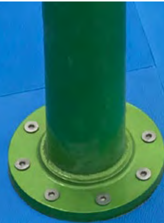
STAINLESS STEEL FOOTING BASE INSTALLATION
